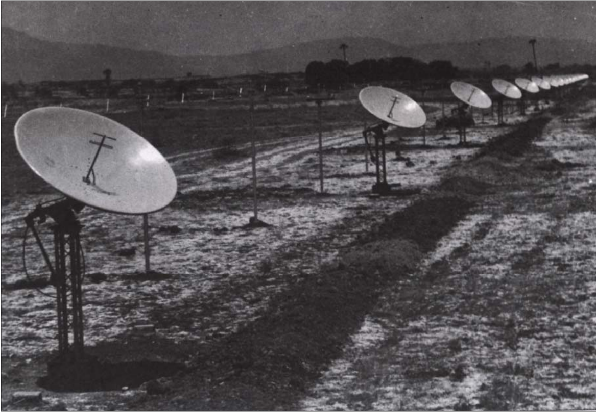
Figure 15: View of the east-west grating array consisting of twenty-four 6-ft diameter dishes built at Kalyan, near Mumbai, in 1965.
