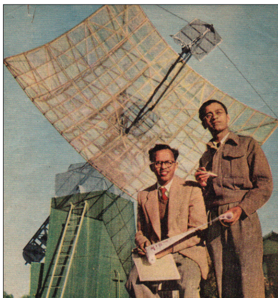
Figure 4: Govind Swarup (left) and R. Parthasarathy (right) in at Potts Hill field station in 1954. At this time, searches were being made for hydrogen clouds in the Milky Way with this 16 x 18 ft ex-radar antenna (after Illustrated Weekly Times of India , 14 September 1954).
