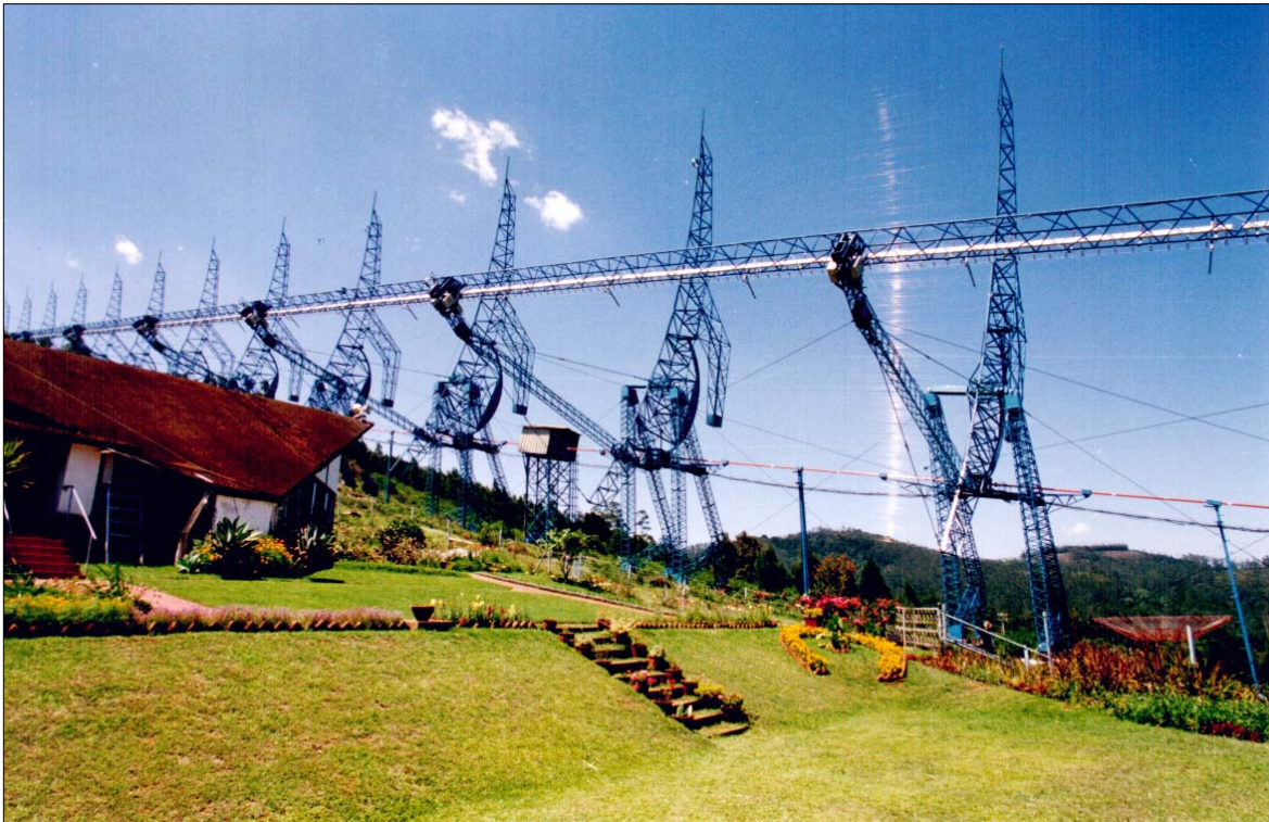
Figure 17: Another view of the Ooty Radio Telescope; reflections of sunlight by 1,100 stainless steel wires are seen on the right.
