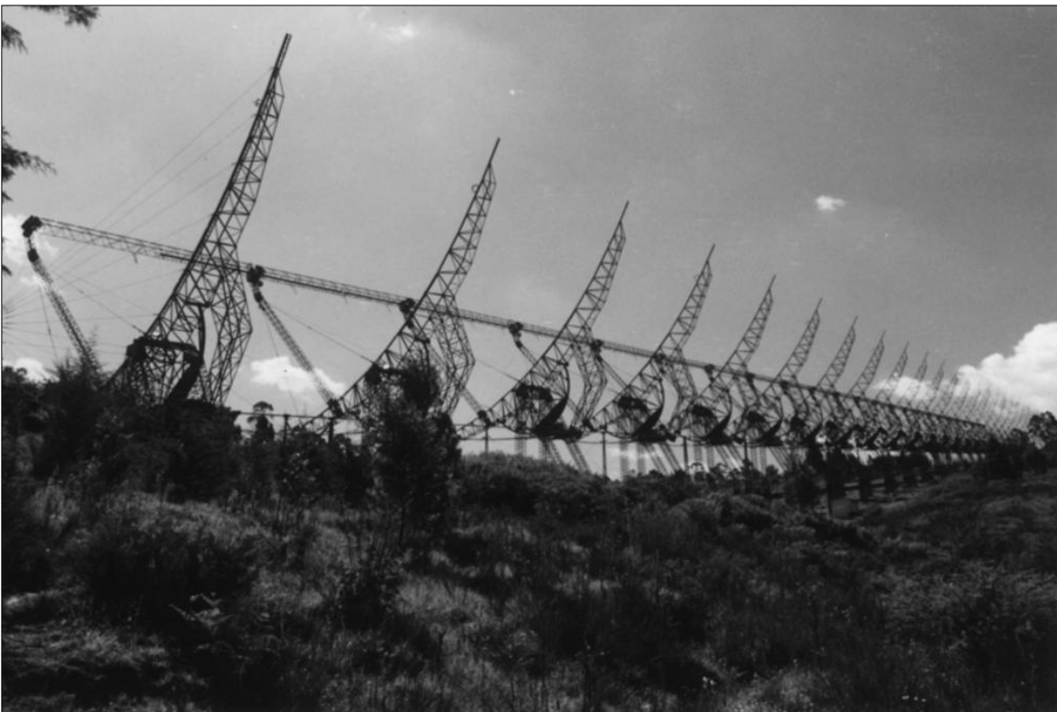
Figure 16: The Ooty Radio Telescope, consisting of the 530 m long and 30 m wide cylindrical parabolic antenna placed along a north-south sloping hillside at an angle of 11.3^\circ so that its axis of rotation is parallel to that of the Earth.
