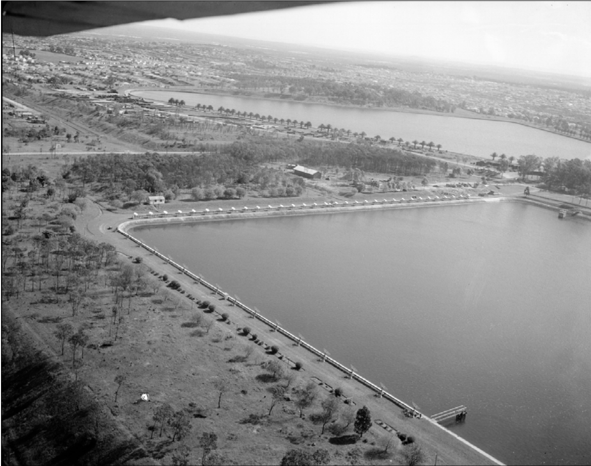
Figure 6: View looking southwest across the two Potts Hill water reservoirs in 1953, showing Christiansen's solar grating arrays along the banks of the eastern reservoir. The E-W array consisted of thirty-two elements and the nearer N-S array just sixteen elements (ATNF Historic Photographic Archive: 3475-1).
